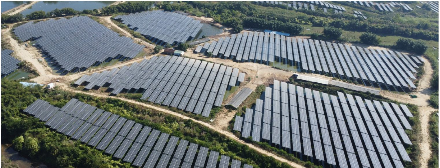
Huizhou Solar Farm (140 MWp)
