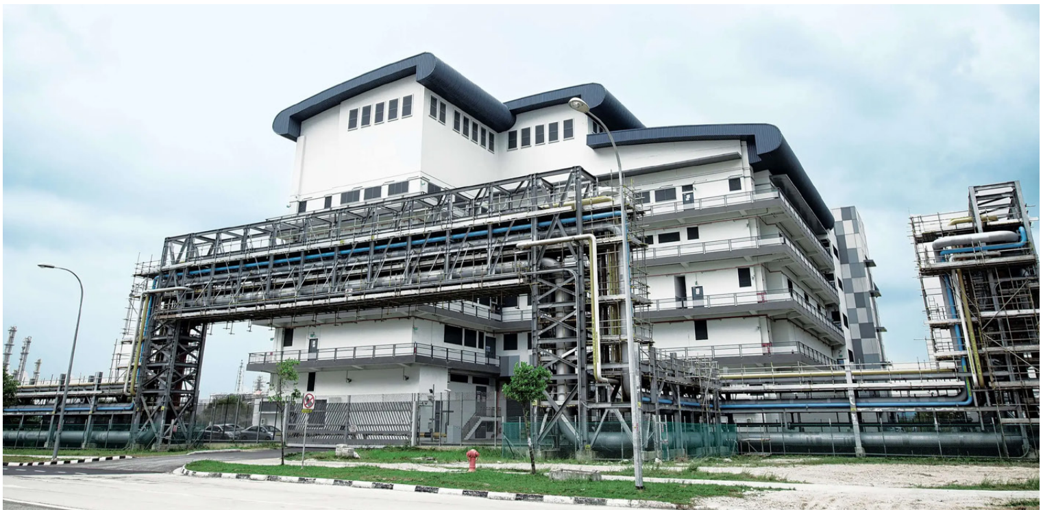
Jurong Island substation. First substation with solar panels installed.
